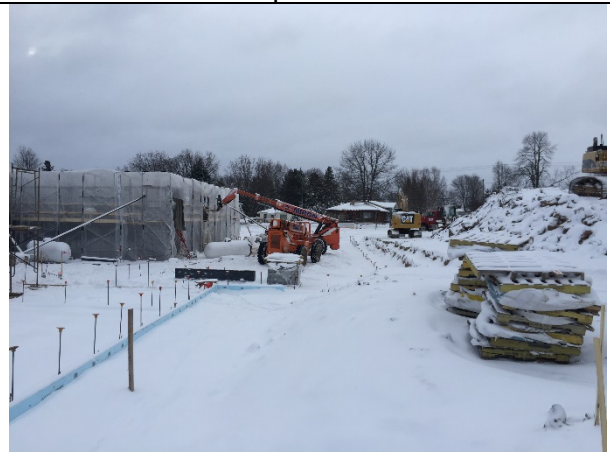
Thomas Jefferson 02/03/2016 Winter conditions return, project continues.
