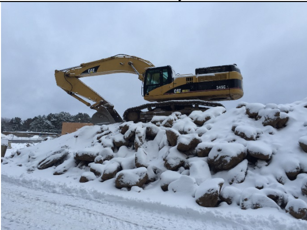
Thomas Jefferson 02/03/2016 Excess material loaded/hailed offsite.
