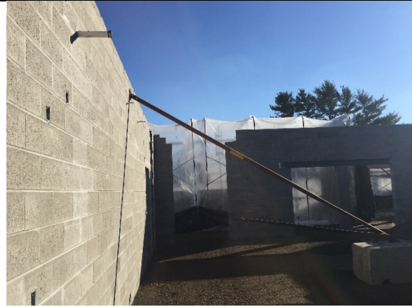
GD Jones 02/01/2016 Masonry walls going up rapidly.
