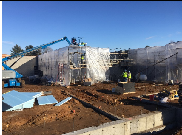
Thomas Jefferson 02/01/2016 Foundations complete on main addition.
